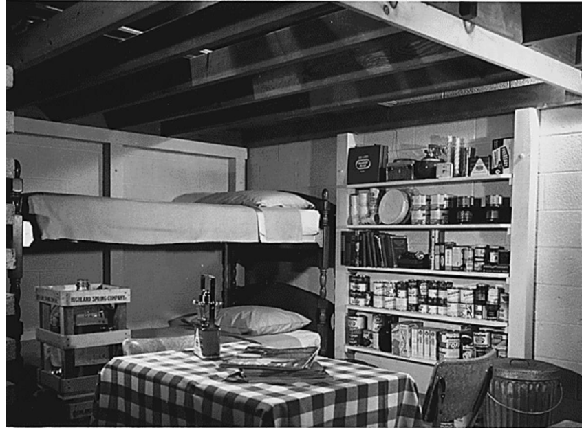
Dual purpose fallout shelter in the basement of a house
