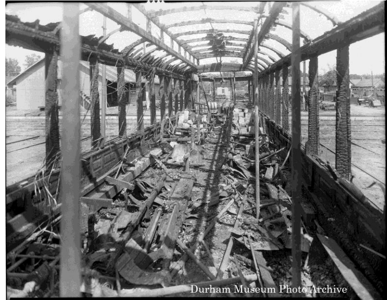
Interior of streetcar damaged in 1935 strikes
