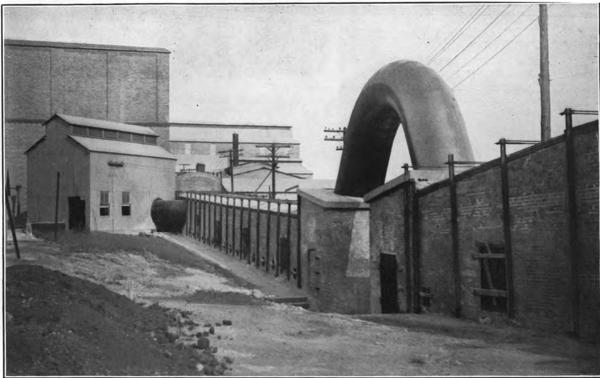
PLATE 15.—FLUE AND BAG HOUSE SYSTEM.
